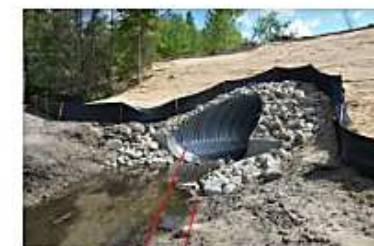
Figure 42: Poor practice, do not use smaller multiple pipes; they can create a barrier to fish passage.
