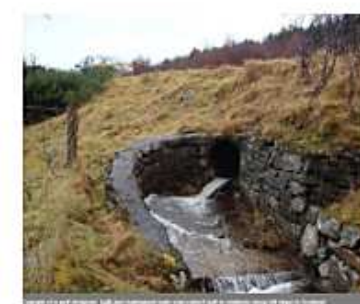
Figure 41: Good practice, use a single large culvert for crossings that maintains the natural channel width.
