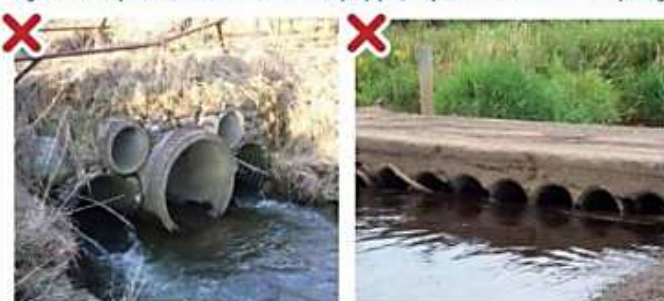
Figure 42: Poor practice, do not use smaller multiple pipes; they can create a barrier to fish passage.
